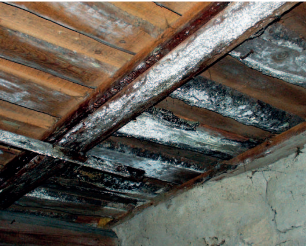
FIGUR 1 Muggsopp i kjellertak pga kondens. MYCOTEAMS BILLEDARKIV
